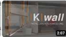
Rough slab to rough ceiling IKIwall installation
